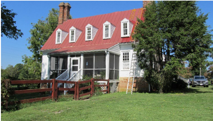
Front view of Sweet Hall which faces the water
